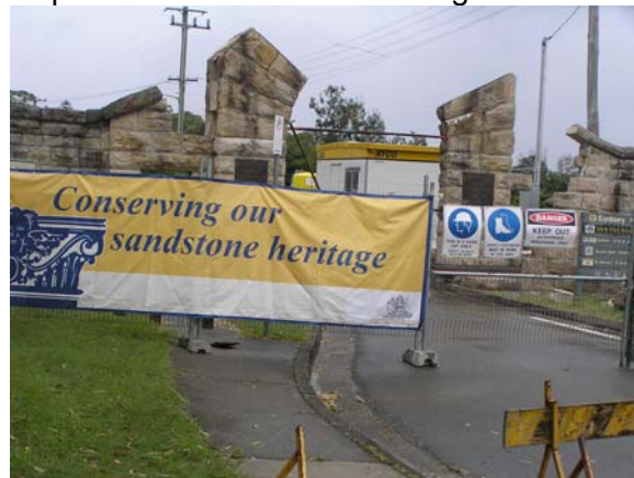
Reconstruction of Arch in February 2008.
